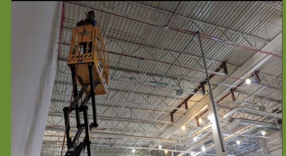
USACE - DESIGN - BID - BUILD B1717 FREEZER CONSTRUCTION AT FORT BLISS
